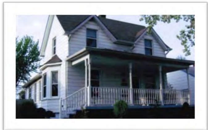
505 E. Chesterfield, Built 1903
