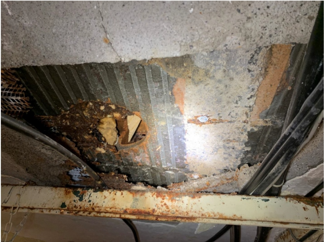
Figure 6. Inspection Opening 5. The only opening where the joist concrete along the bottom edge was sound.
