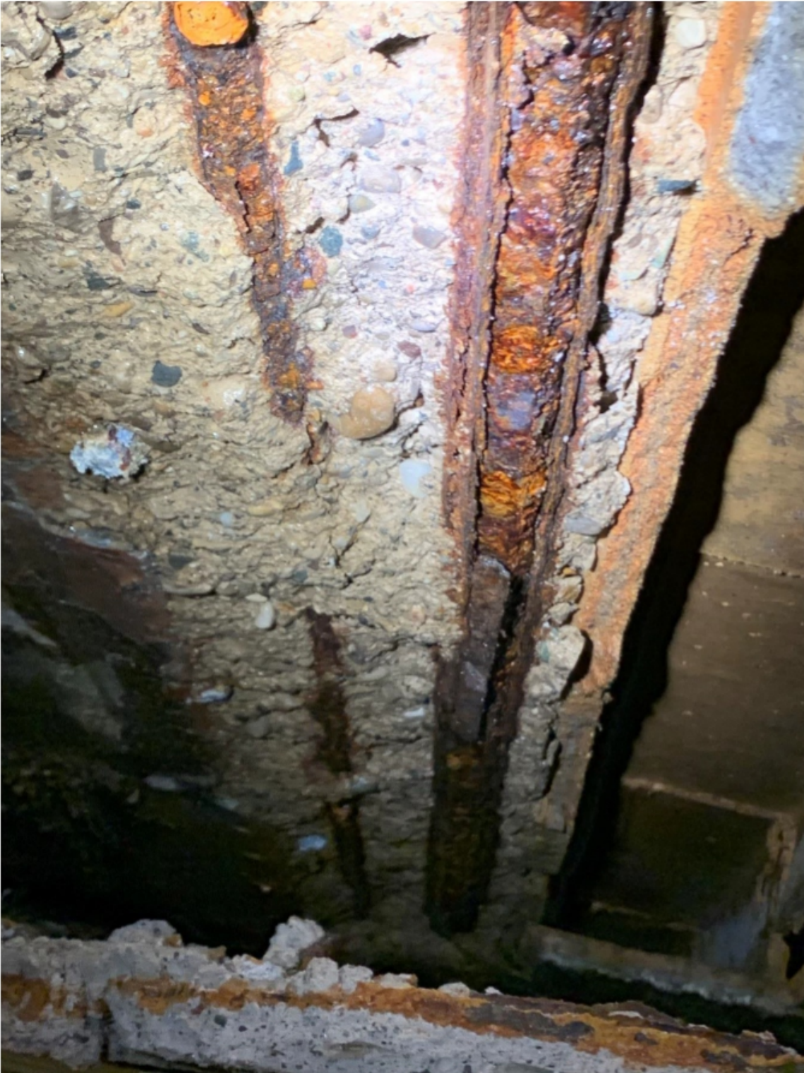
Figure 4. Inspection Opening 3. Heavily corroded bar with section loss.
