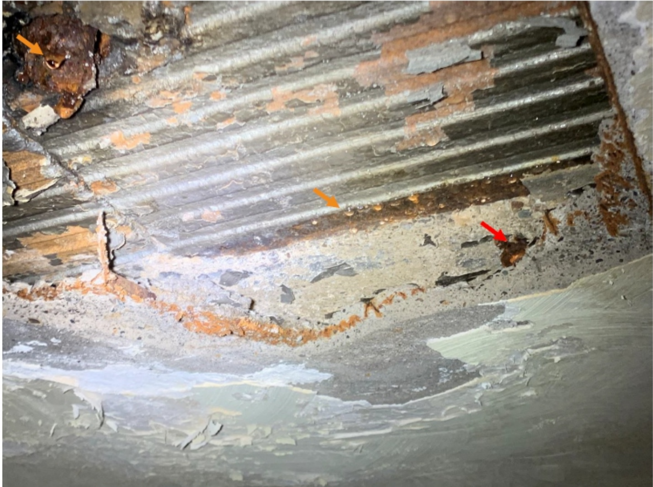
Figure 3. Inspection Opening 2. Red arrow points to exposed corroded bar post sounding and breaking free loose concrete. The orange arrow points to formed water droplets.
