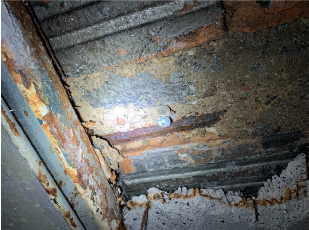
Figure 2. Inspection Opening 1. Corroded octagonal bar.
