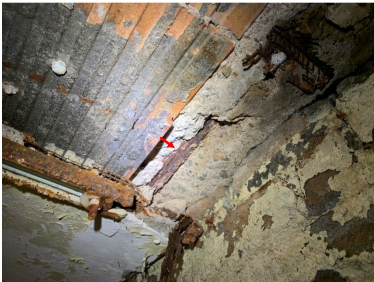
Figure 5. Inspection Opening 4. Typical distressed conditions. Red arrow points to corroded reinforcing bar.
