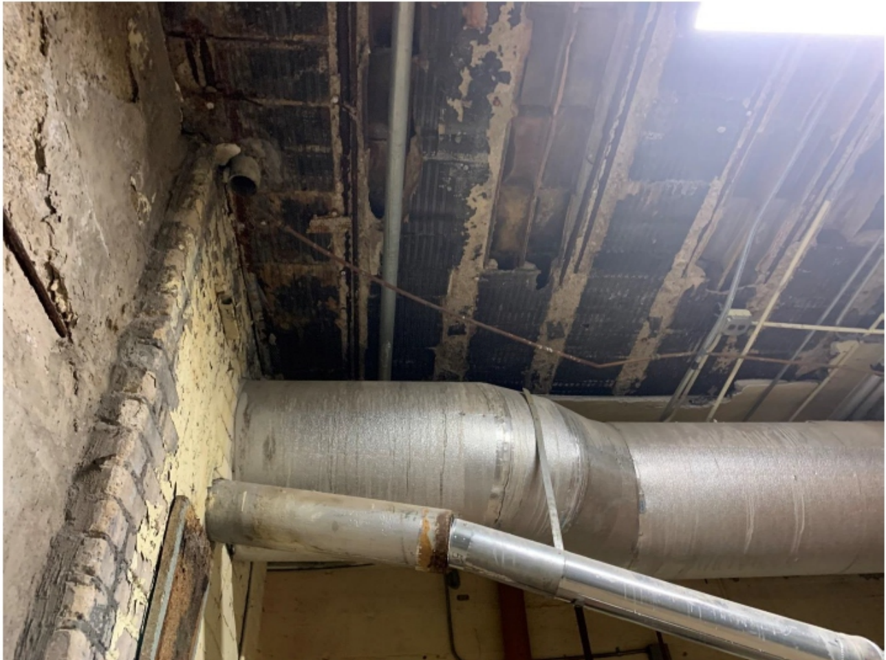
Figure 1. North end looking east above stairs. Area where the ceiling finishes fell. Note the bottom webs of the clay masonry are broken and missing.
